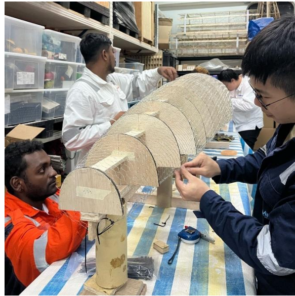
Figure 9-9 Laying chicken wire
